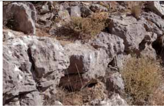
RUBBLE WALLING Round and radiate rubble walling contains the ground. This walling is more obvious in Soroi that are almost destroyed due to human interference.
